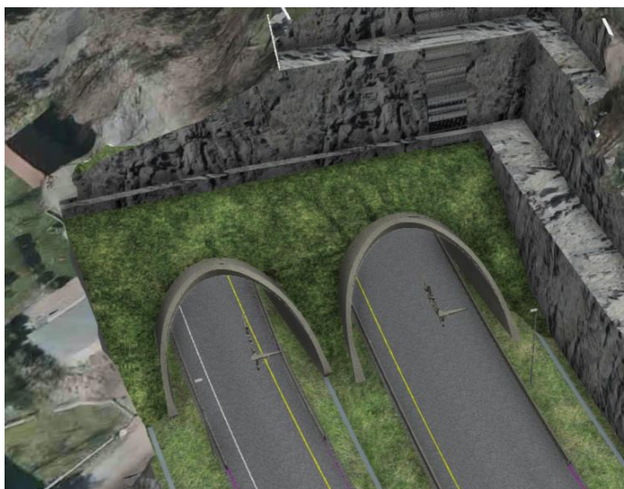
Figur 6-17: Tunnelportaler i Vige.
